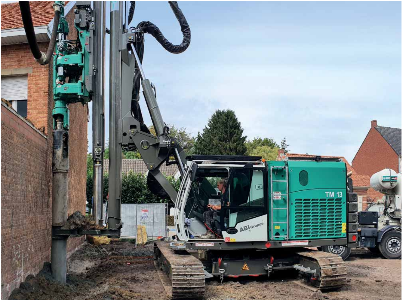
Installation of secant pile wall with a minimum distance to the existing structure using a VDW auger drive. The drilling and concreting is carried out in one continuous step, after drilling down concrete is pumped during withdrawal.
