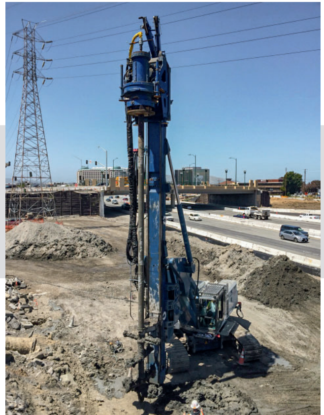
Drill rig in a short leader mast application with limited headroom: The required depth is achieved by installing additional pipe sections on the mixing rod.
