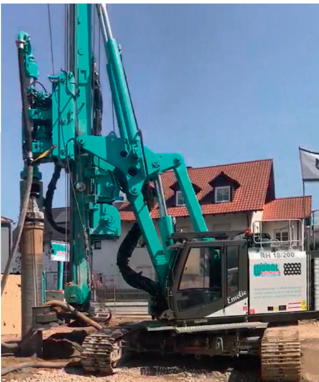
DELMAG drill rig during VDW drilling: The pile is created in a single pass. Immediately after reaching depth the concreting takes place and continues during the extraction process.
