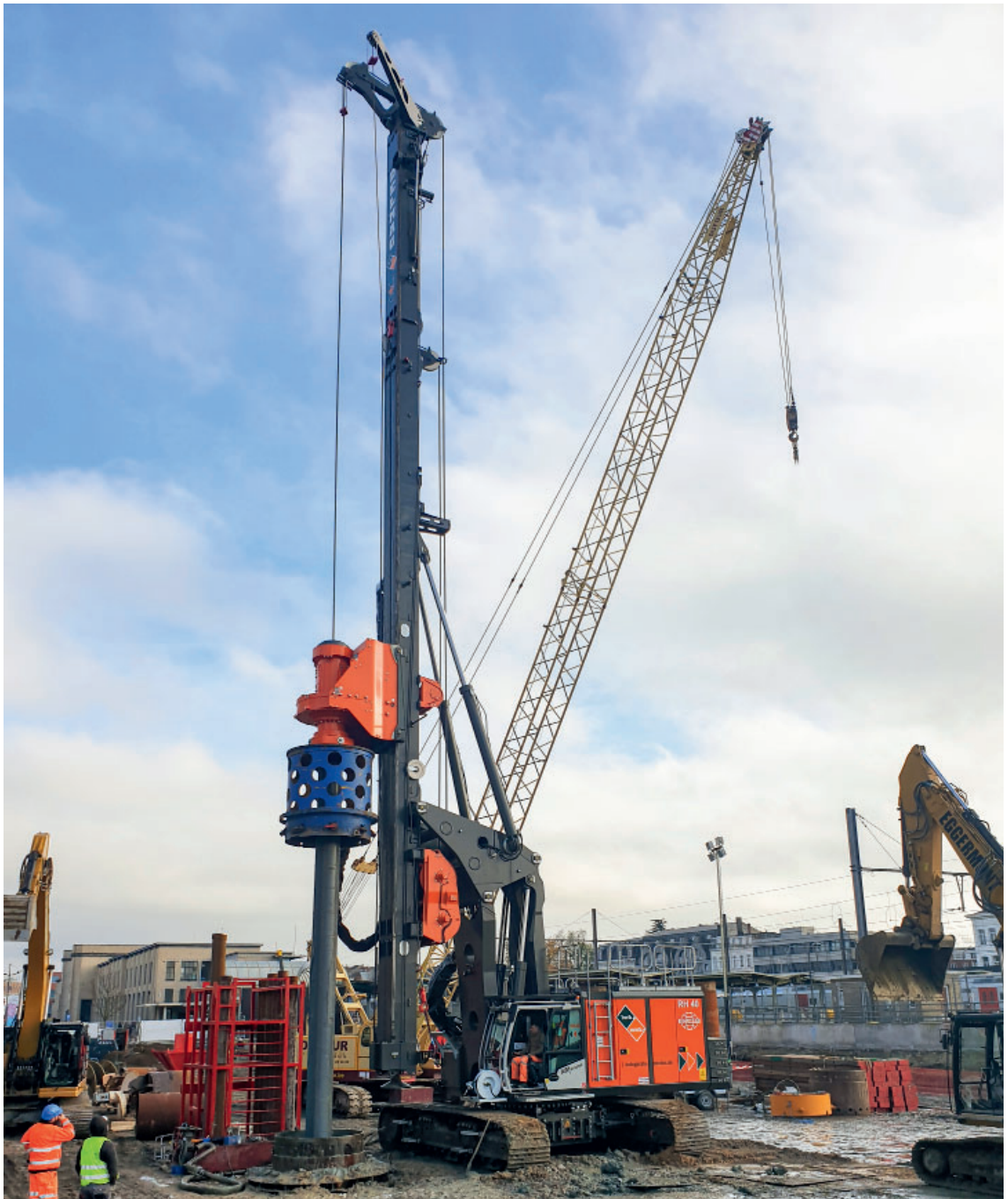
The biggest model of the DELMAG rotary drill rigs built on an ABI T110 carrier for the production of drilled piles with a diameter of 1800 mm and to a depth of 40 m using the Kelly drilling method.
